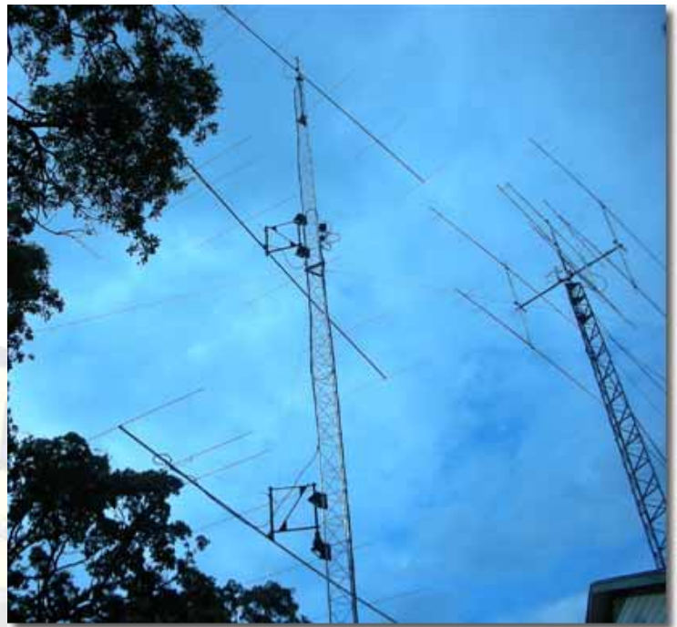
The Texas sized stack of Yagis for 6 meters (left), the 2 meter through 2304 MHz tower, (right).
