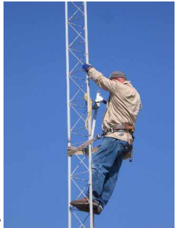
#4 remove tower sections with jack!
